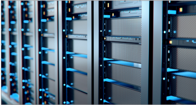
Setup for continuous automated testing
